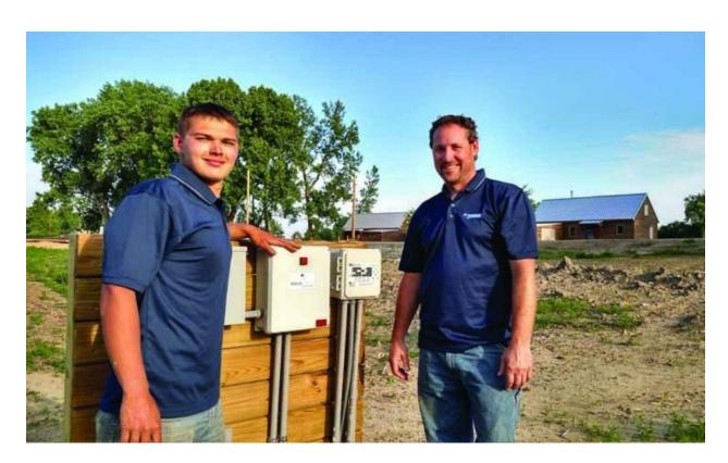
Ray Tebo, right, and Tayler Layne, of New Excavating Technology Inc., finish installing one of the Aquaworx panels for a lift station and a Bio-Microbics panel that controls the MBR systems at Giant Goose Ranch. Each panel can download data to a USB drive, allowing periodic readjustment of the system to more closely match demand.
